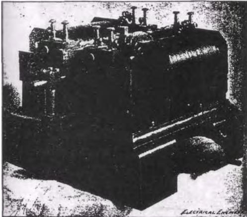
At the left is a photo of Tesla's earlier oscillator, which was unfortunately destroyed by fire in 1895. Projecting at its bottom right is a tube for connection of the compressed air line. Across the top are electrical posts to carry exciting current to the windings (around the outside), and from which generated power is extracted.
